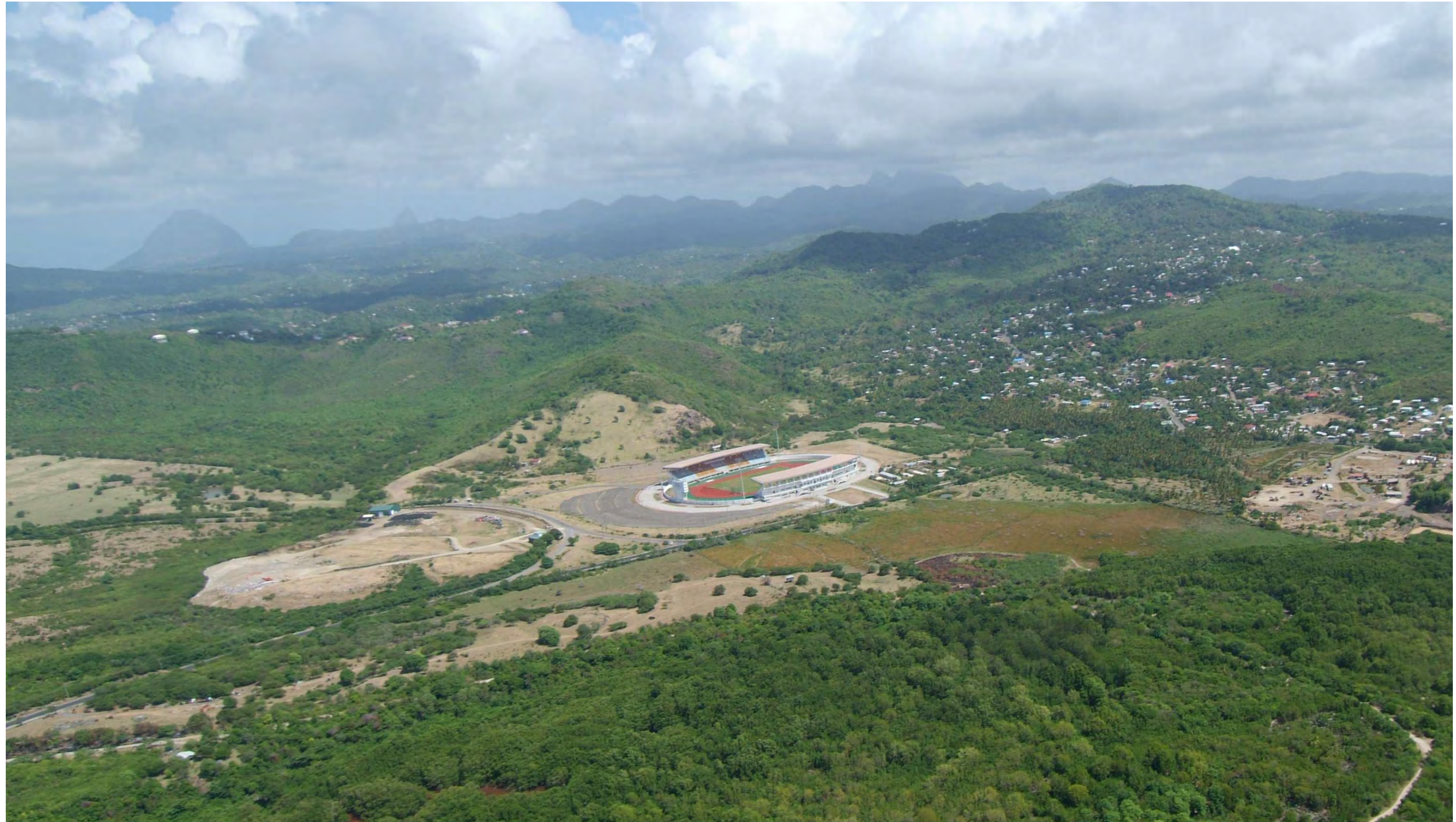
VIEUX FORT NATIONAL STADIUM PHOTO
